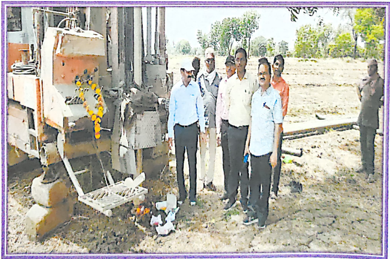
Image 16: Construction of Bore well in the research field
