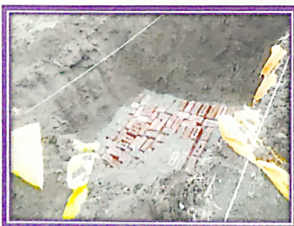
Image 5: Sand and bricks layer laid at bottom of pit
