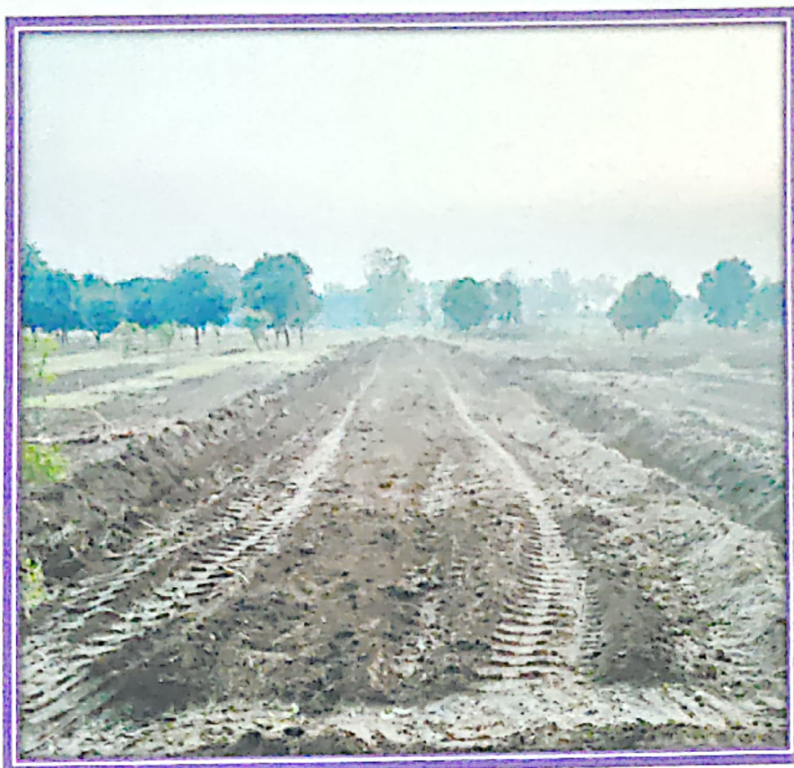
Image 11 : Laying of road at research field
