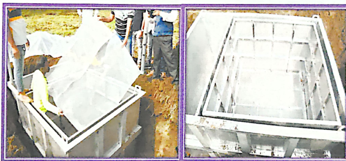
Image 7: Installation of outer tank in pit
