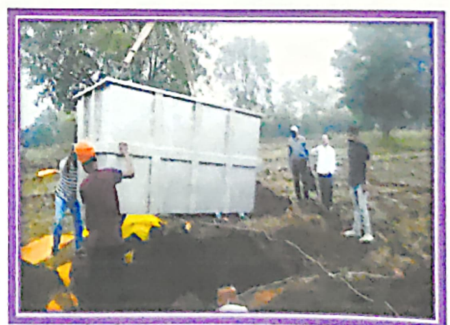
Image 6: Installation of outer tank in pit
