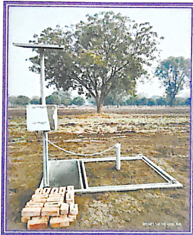
Image 10: Installation of solar panel
