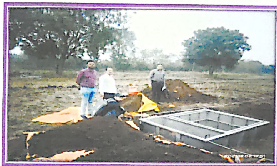
Image 7: Installation of outer tank in pit
